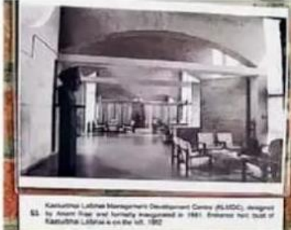
Karambhai Lalbhai Management Development Center (KLMDC), designed by Anant Rao and formerly inaugurated in 1981. Entrance to the building of Karambhai Lalbhai & on the left, 1982
